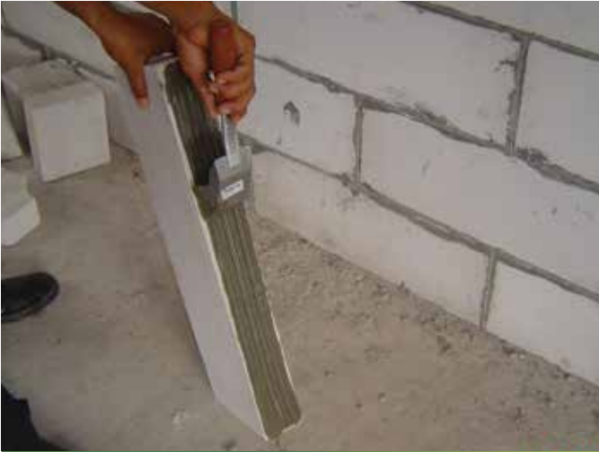
Procedure for bricklaying
